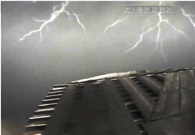
Fig. 4.6-2: Lightning striking immediately in front of the weather station
